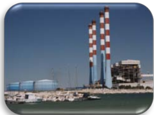
Start of Martigues CCG (France)
